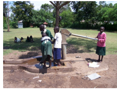
Odiinya students using safe water from a drilled borehole
