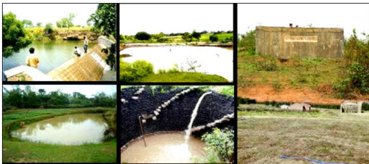
Figure 3.16. Types of rainwater harvesting (stone and earthen check dams), storage (tanks) and groundwater recharging (wells) structures.
