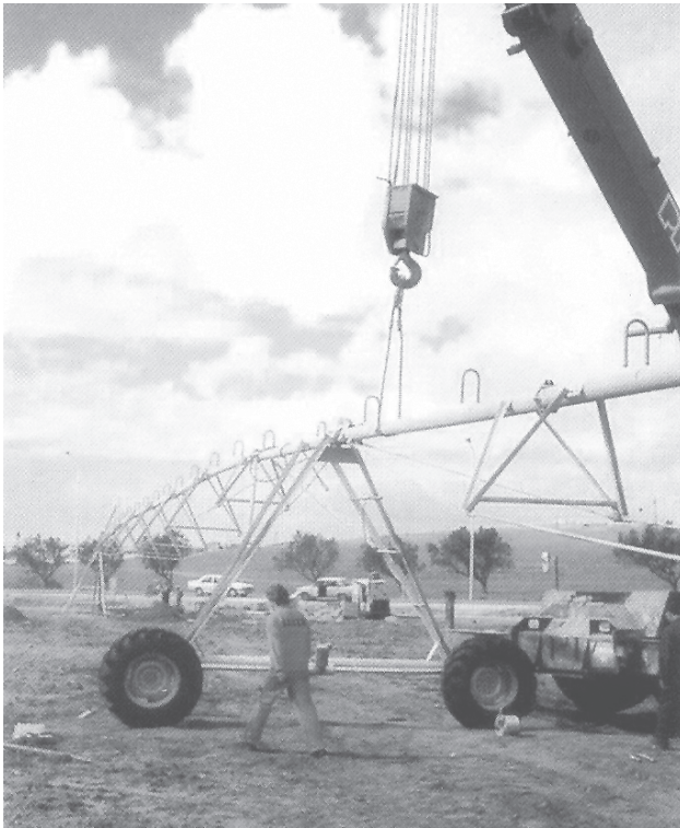
FIGURE 10.7 - The erection of a center pivot.
