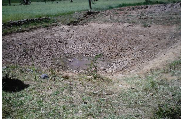
Figure 2: Pond compacted with clay and stone riprap
