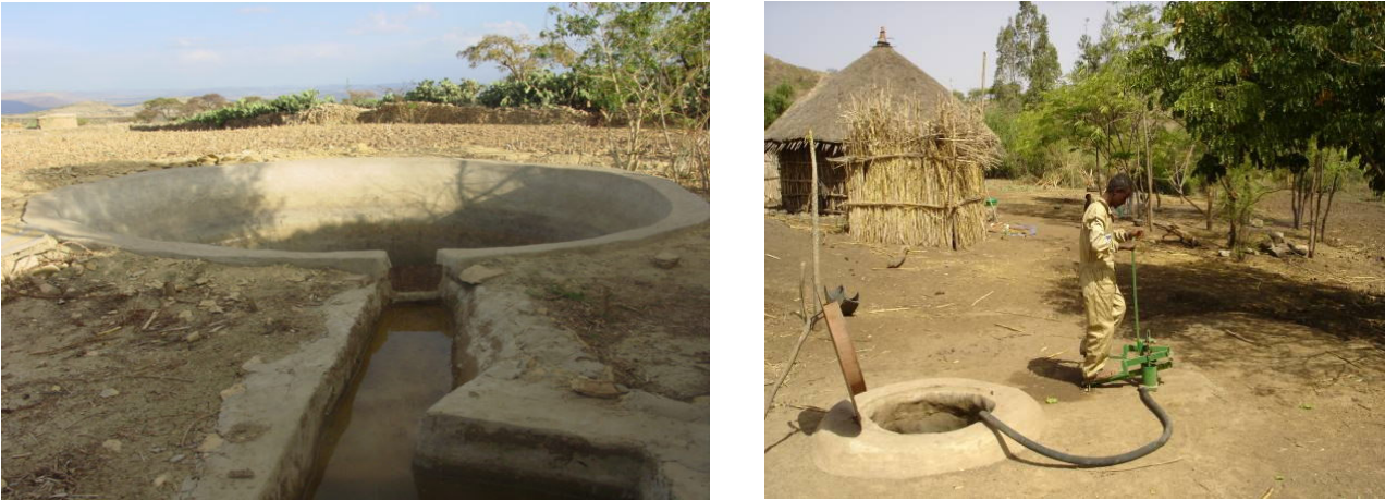
Figure 5: Household underground tankers of different shape
