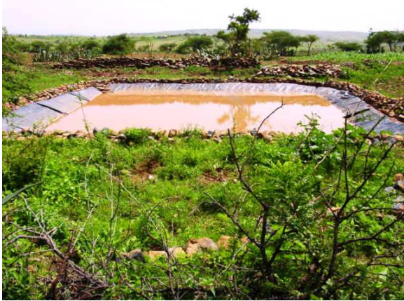
Figure 1: Pond with geo membrane lining sheet
