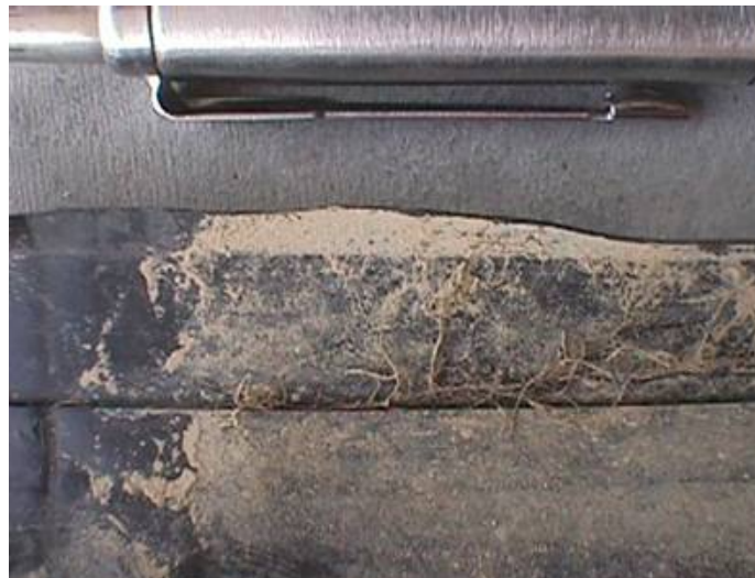
Figure 13. Root intrusion
