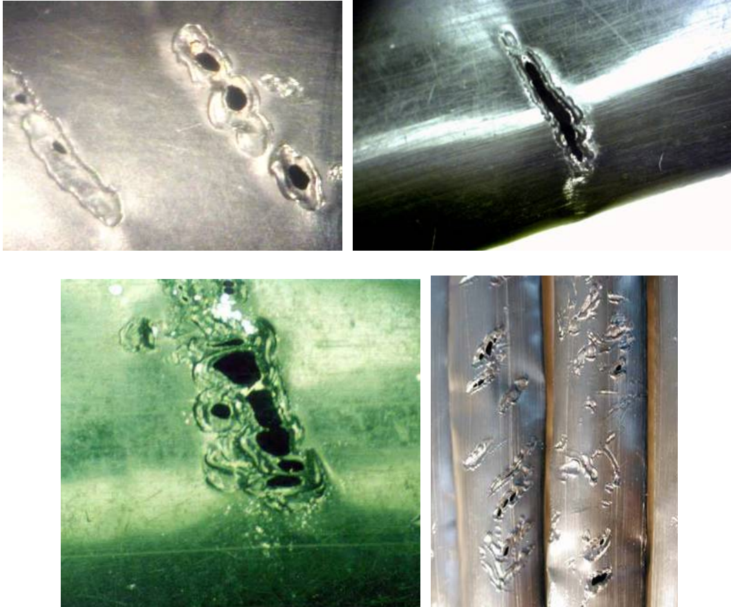
Figure 20. Damage due to the “magnifying glass effect”. Note the rounded edges.
