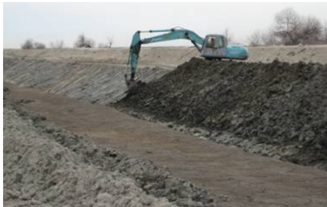
Figure 3. James ID Main Canal during side compaction
