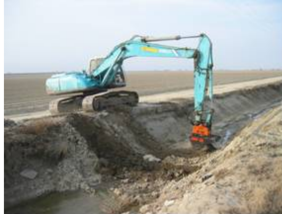
Figure 6. Compacting the sides and bottom of Lateral H at James ID
