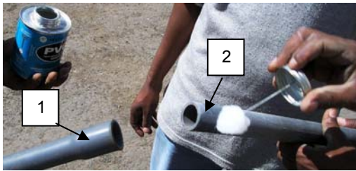
glue the pipes together
