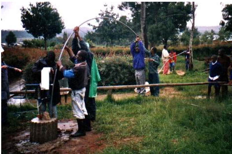
Installing the guide box with rising main and rope.
