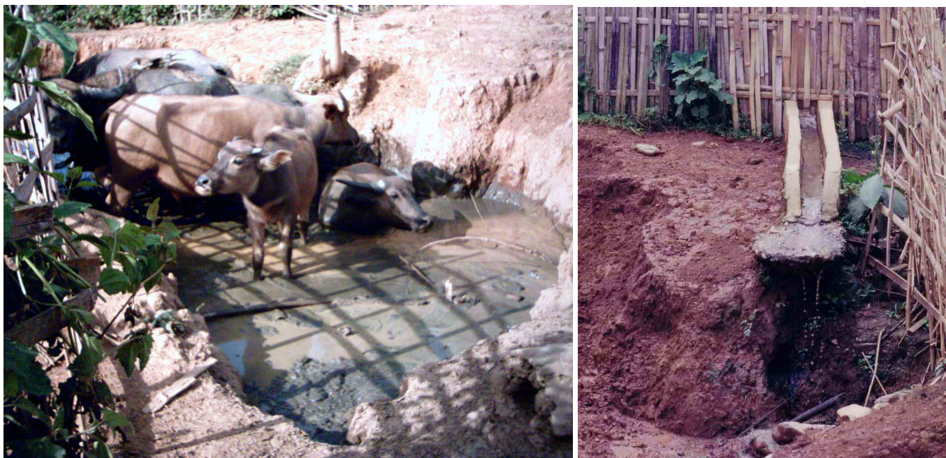
Fig.6 : Pond and gully and formed at the level of a tapstand drainage.
