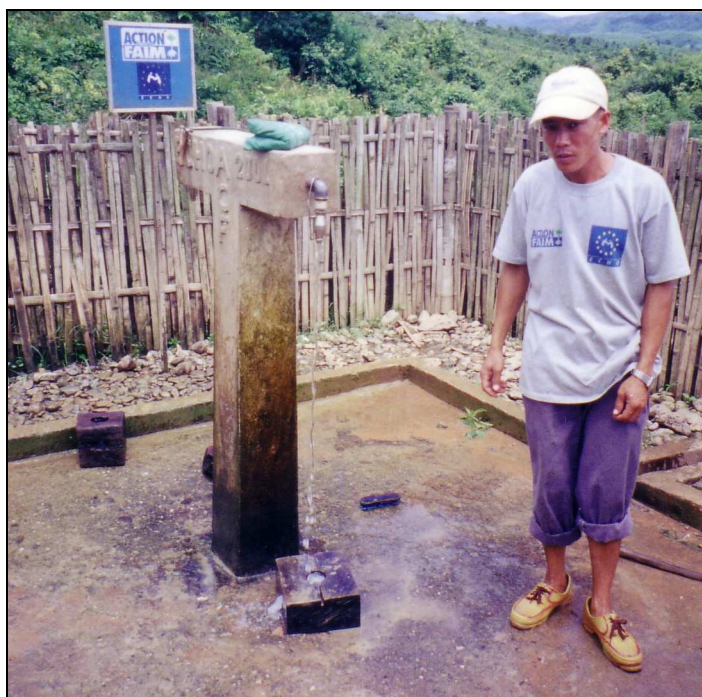
Fig.15: Example of tapstand . A piece of wood is used to avoid erosion of concrete and splashes of water
