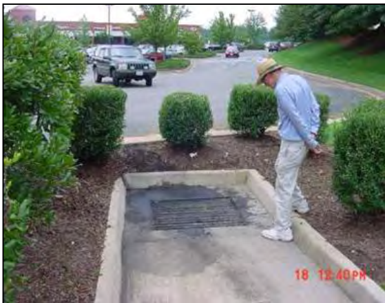
Figure 7: Understanding the plumbing: measuring pipe inverts at drop inlets.
