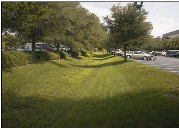
Figure 1: Dry Swale
