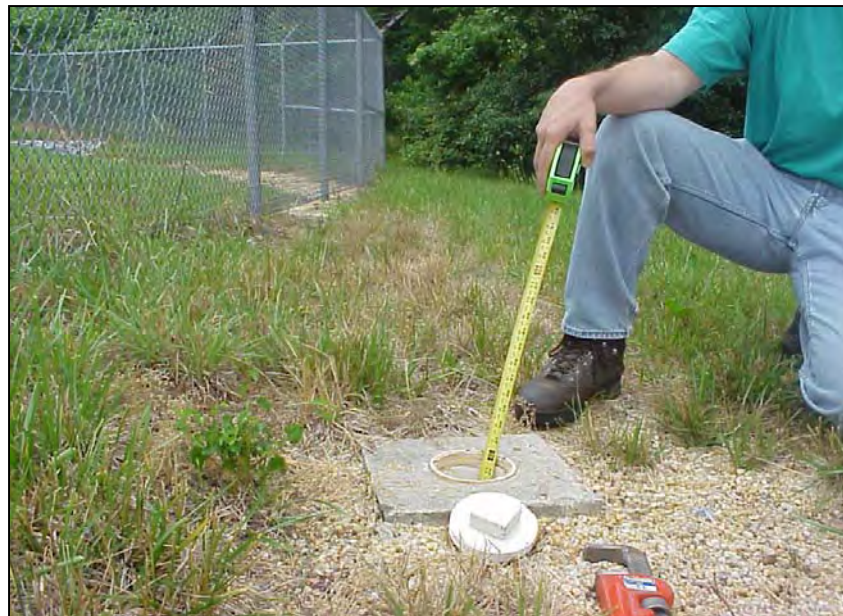
Figure 4.19: A final inspection is needed to identify and correct any problems before as-built certification
