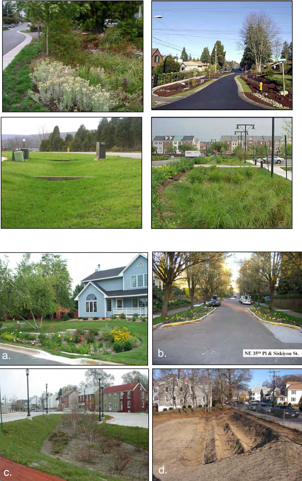
Figure 3: Innovative street retrofits include: curb cuts to rain gardens (a), surface bioretention in traffic calming measures (b), larger bioretention pocket in multi-family residential (c), and curb cuts to cascading bioretention cells (d).
