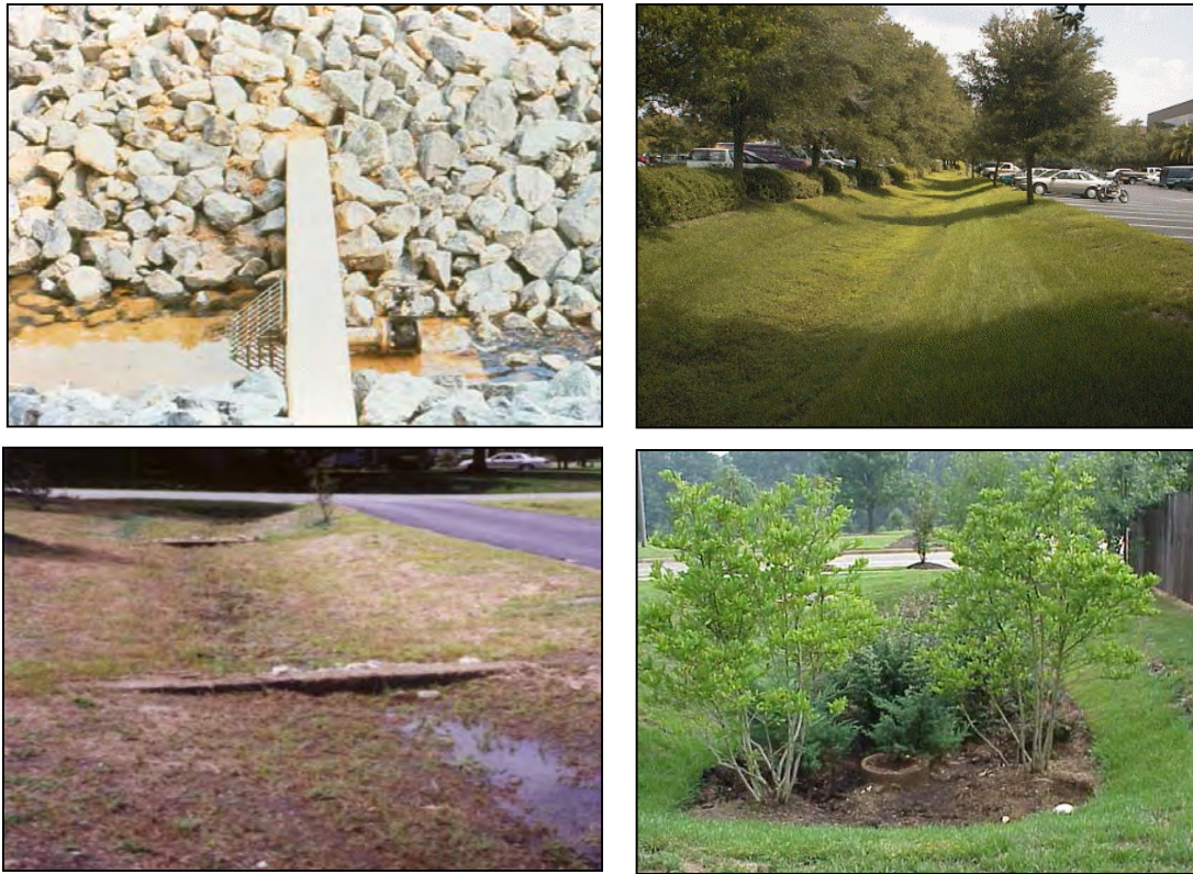
Figure 10: Four examples of conveyance retrofits.
