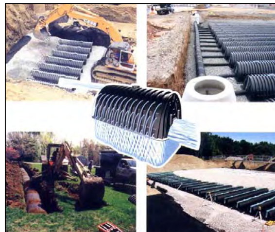
Figure 4: Where soils permit, infiltration galleries can be used to treat stormwater underground.
