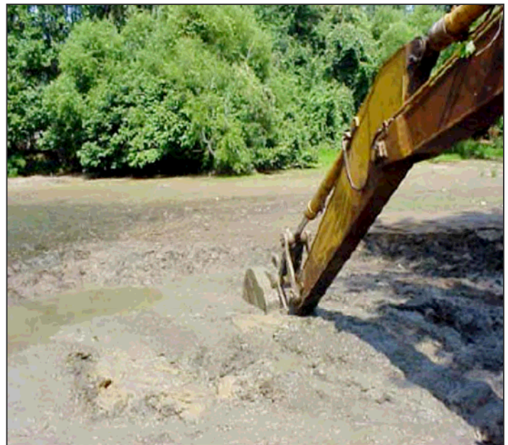
Figure 11: Dewatering is needed to excavate bottom sediments.
