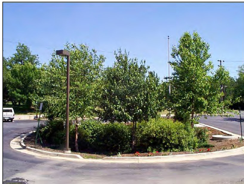
Figure 1: Bioretention created in a parking lot turn-around
