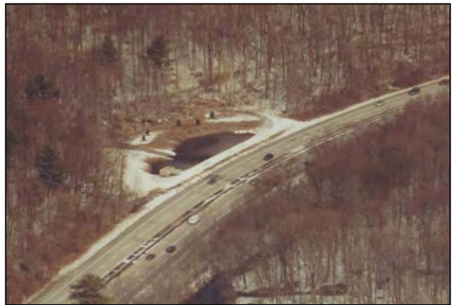
Figure 10: Two examples of crossing retrofits
