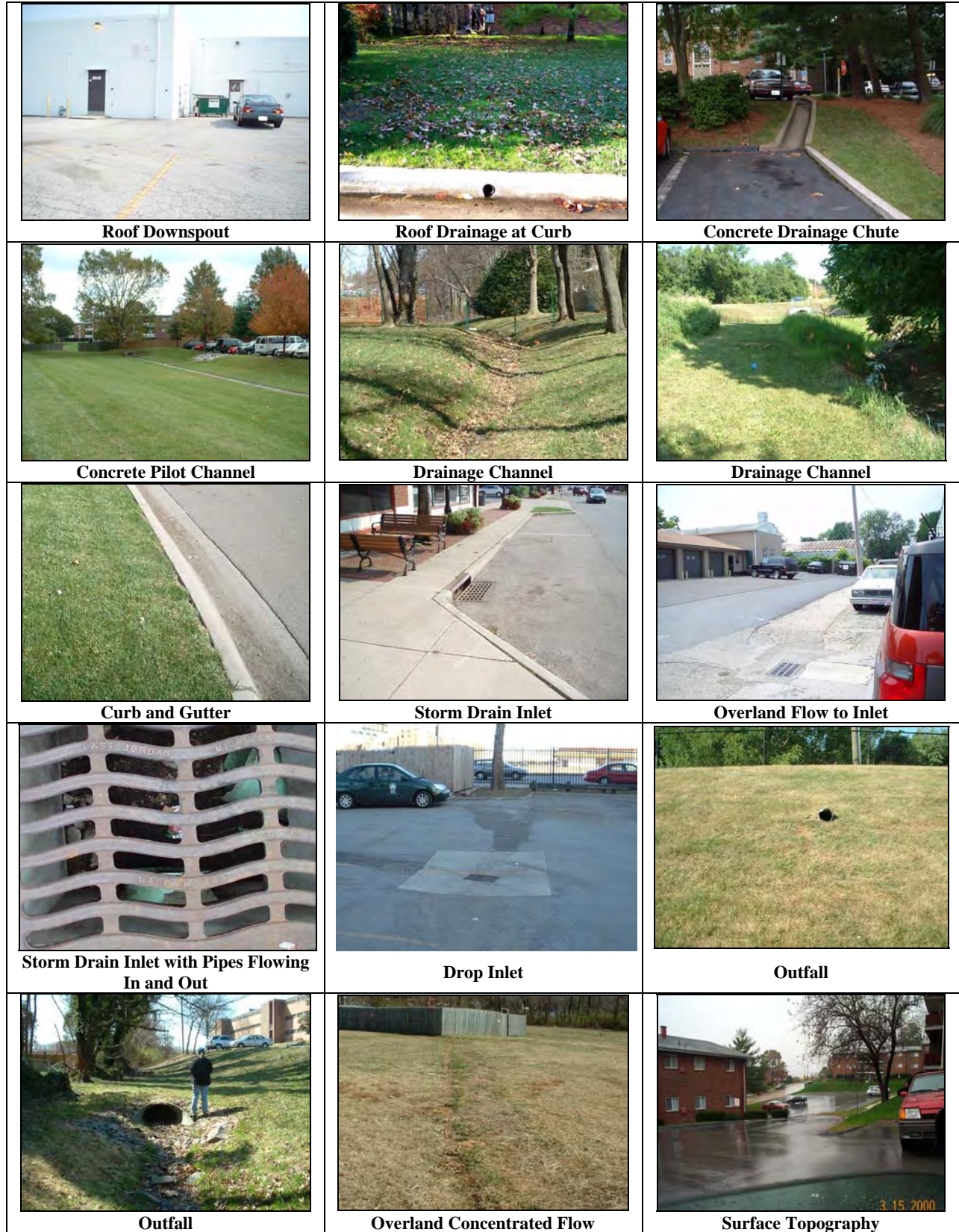
Figure 4.5: Examples of Stormwater Infrastructure Indicators
