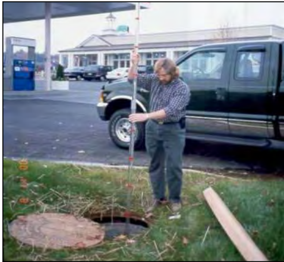
Figure 5: Out of sight means out of mind – make sure inspectors can access underground retrofits.
