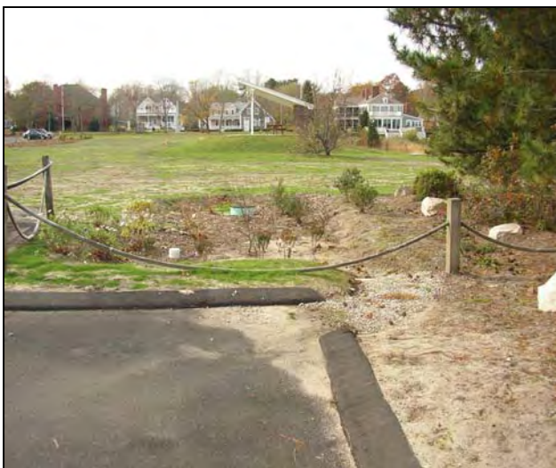
Figure 7: While ponds are most common, larger bioretention areas can provide effective treatment.
