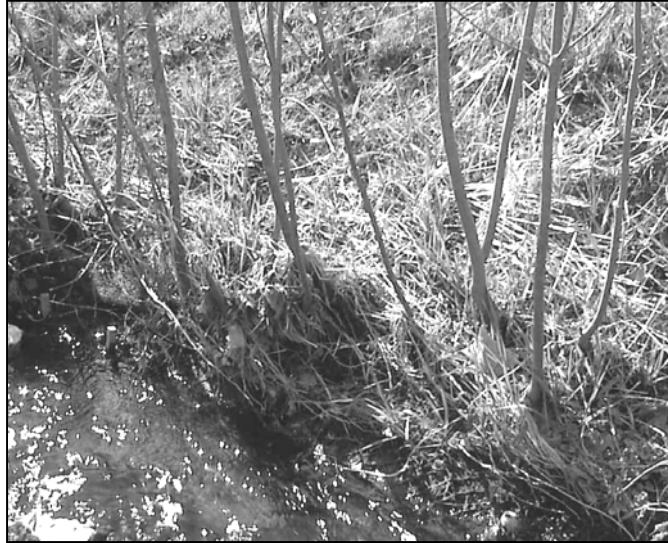
Figure 3: Fascines installed behind a coir fiber roll
