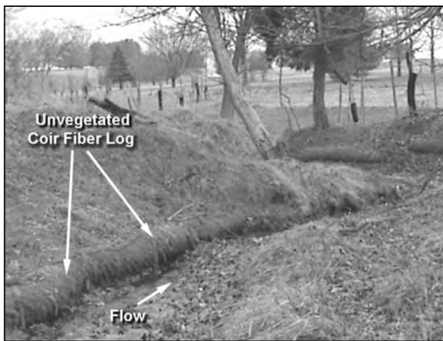
Figure 1: Coir fiber log prior to plant installation
