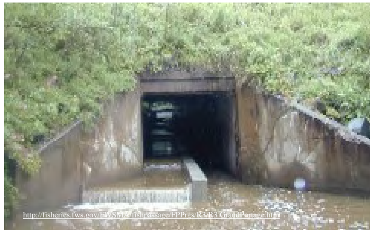
Figure 1: Baffle Step Pool Structure
