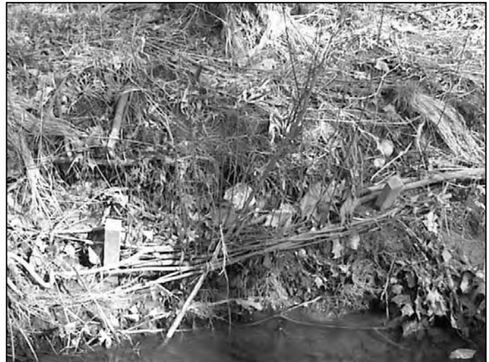
Figure 2: Fascines installed along a streambank
