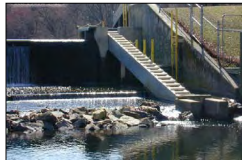
Figure 2: Alaskan Steep pass fish passage structure
