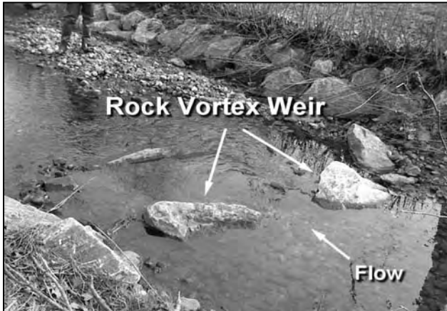
Figure 5: RVW with proper rock spacing
