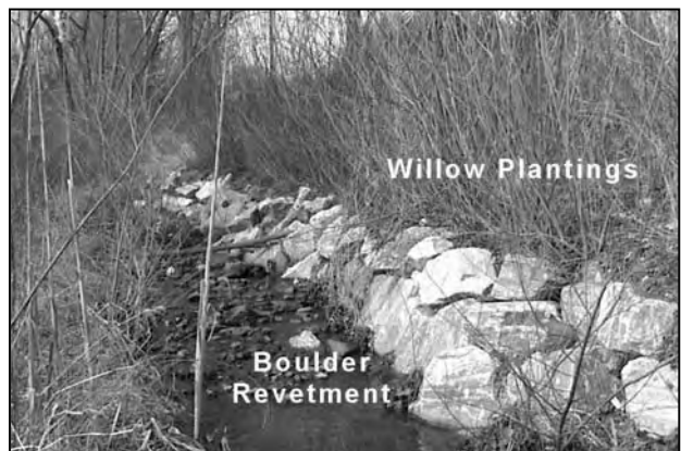
Figure 2: Boulder revetment with willow plantings along an urban stream
