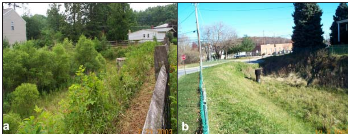
Figure 14: Overgrown Dry Pond (a) and a Well-Maintained One (b)
