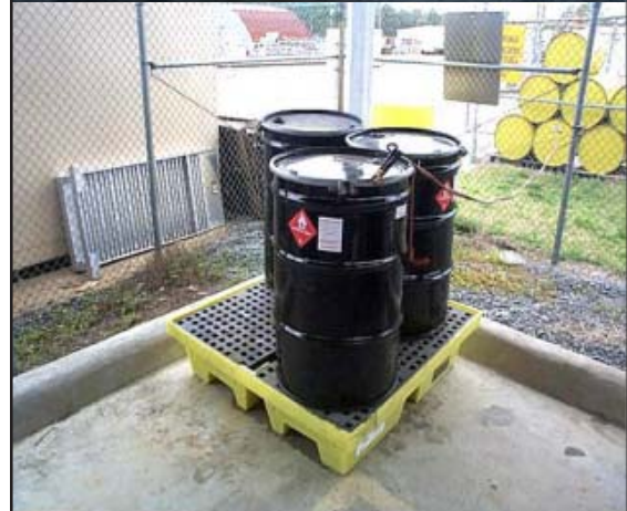
Figure 23: Two Examples of Secondary Containment
