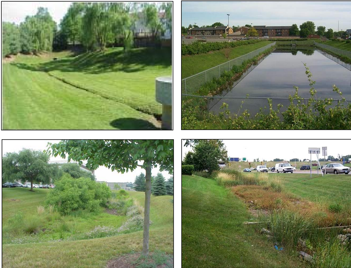
Figure 1. Stormwater management practices include (clockwise from top left) extended detention ponds, wet ponds, bioretention area and swales
