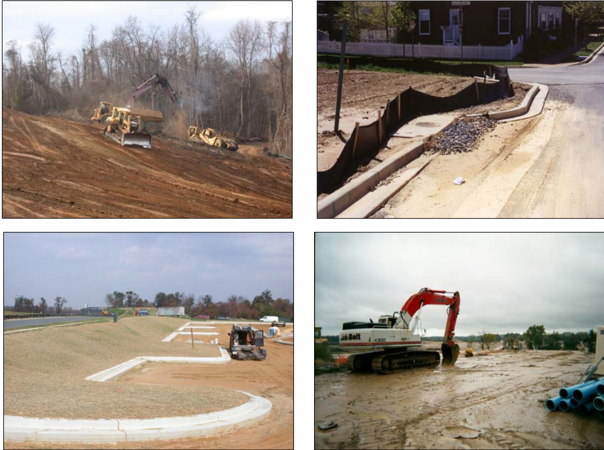
Figure 1. Active construction sites can generate a variety of stormwater pollutants, the most notable of which is sediment.
