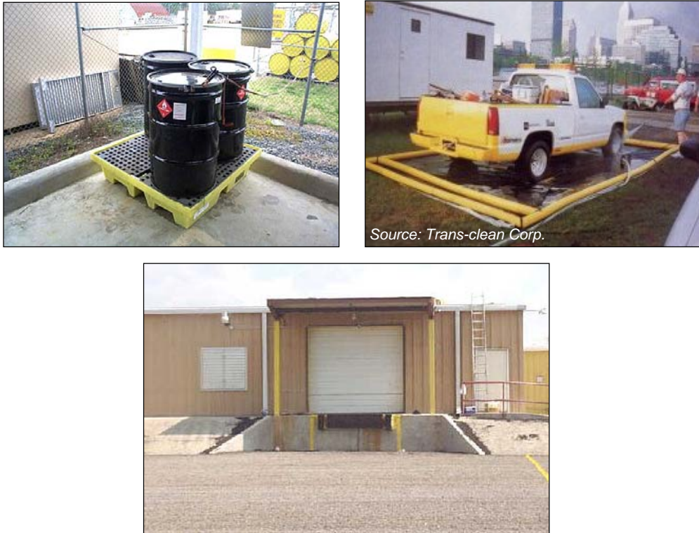
Figure 3: Pollution prevention/good housekeeping practices commonly used at municipal hotspot facilities include (from top left) secondary containment, wash water containment and covered loading/unloading areas.
