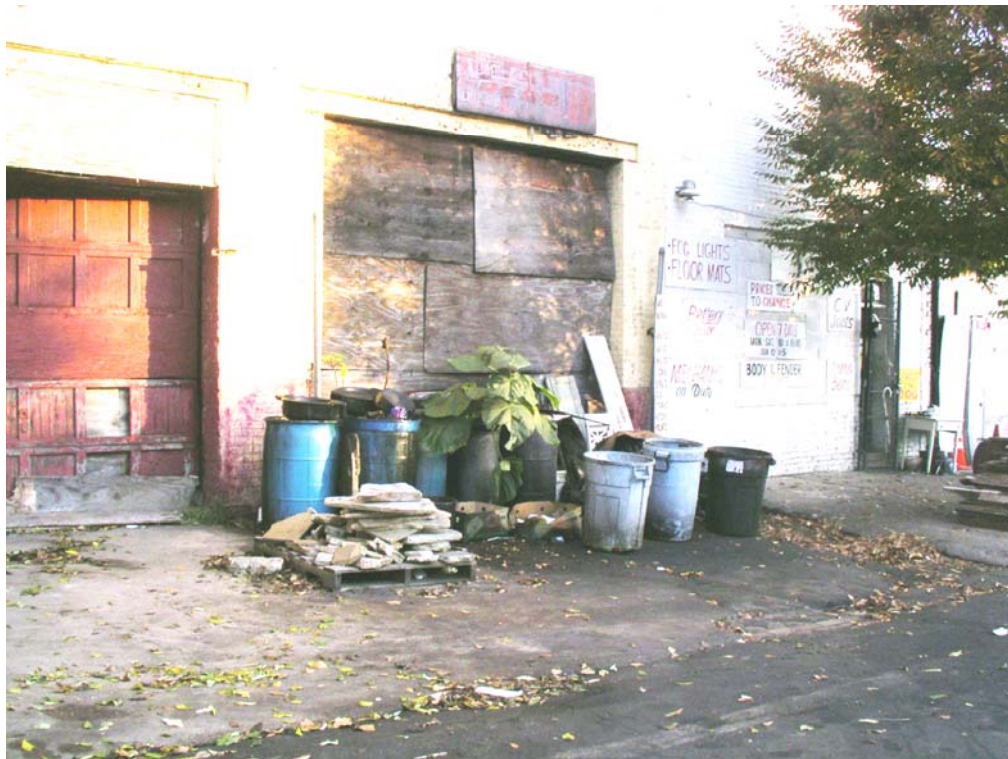
Figure 19: Hotspot Site Investigation
