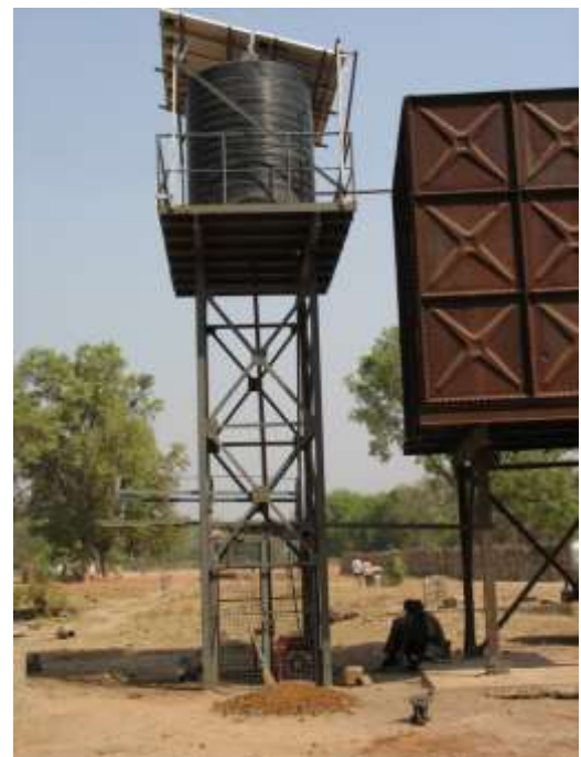
Figure 8: Solar Powered System in Rumbek
