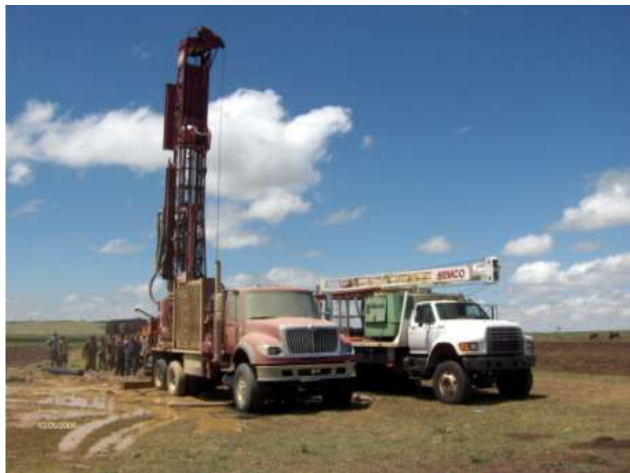
Figure 13: The T3W Drill Rig
