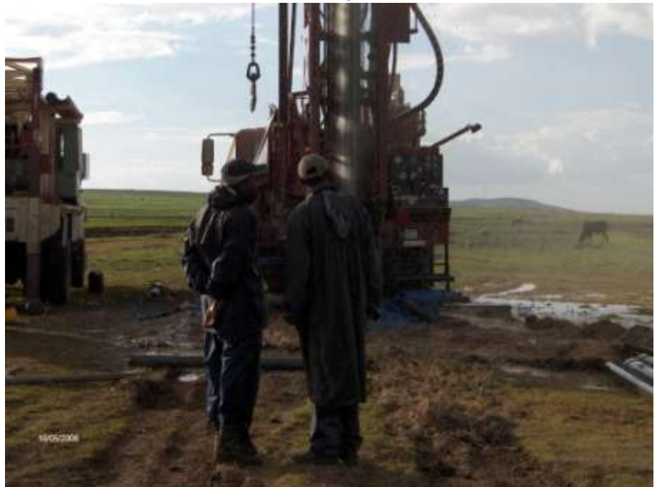
Figure 15: Well Development in Progress
