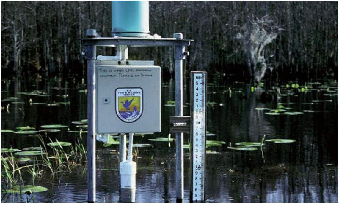
Photo 2.2 Water level monitoring is an essential element of environmental flow management.
