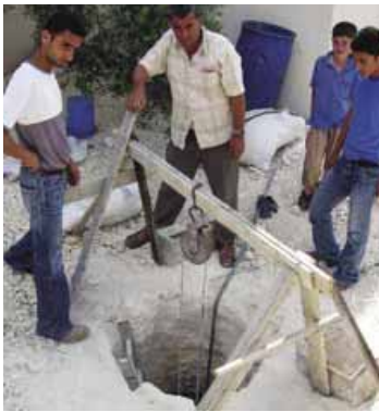
Construction of the well
