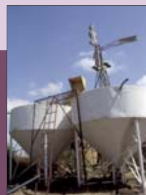
Glass fiber decantation tank
