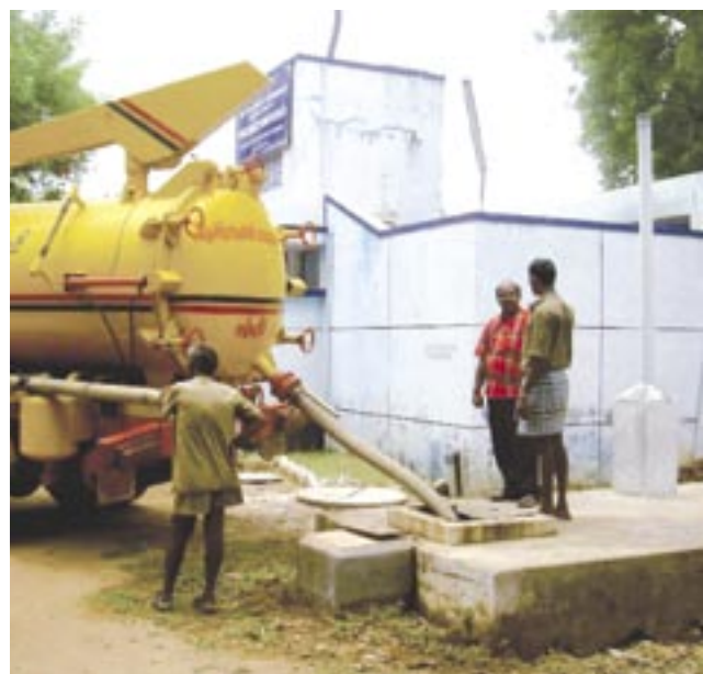
Cleaning septic tank in the slum of TV Kovil
