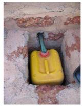
Figure 9. Low-cost solution: 20 L plastic jerrican for urine storage at individual toilet level in Ouagadougou, Burkina Faso (source: E. v. Münch, 2006).
