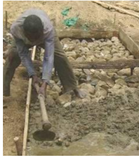
Distributing mortar on top of the ballast
