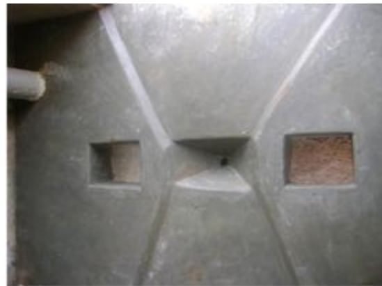
Modulated squatting pan in Kericho Unilever estate
