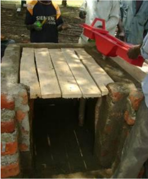
Fixing shuttering timber in the chamber wall
