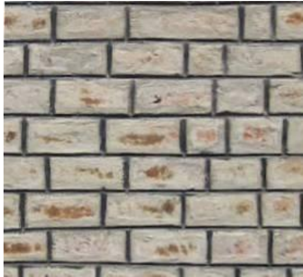
Wall surface after finishing
