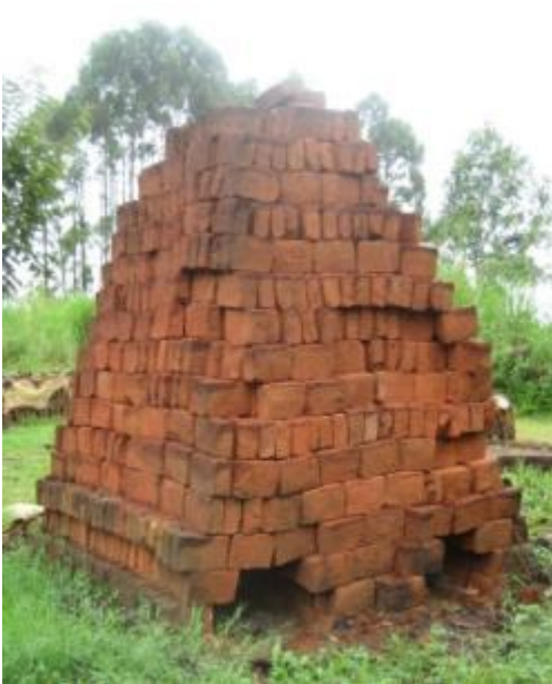
Pile of locally made earth blocks (8 x 6 x 6 inches) in Uganda
