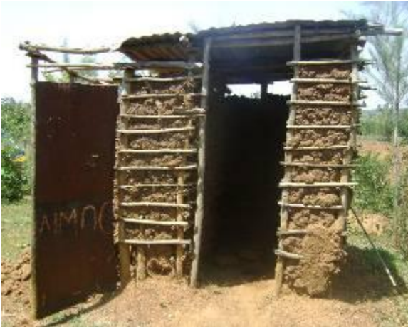
Simple local super structure made from wooden sticks and very little earth near Ugunja
