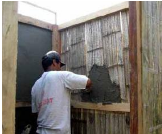
plastering from the inside of the cubicle
