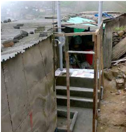
Toilet during the construction without walls
