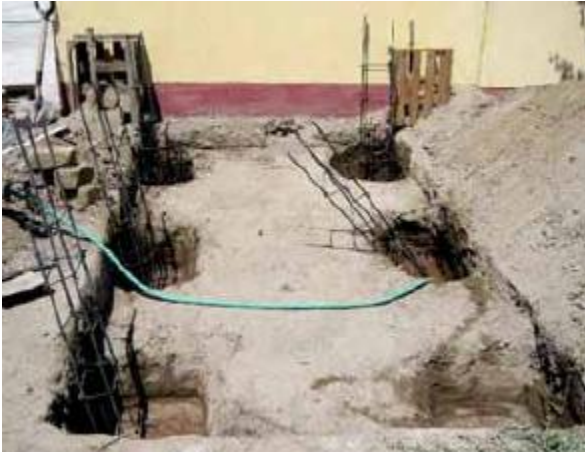
Preparation of the Ferro-cement foundation pillars
