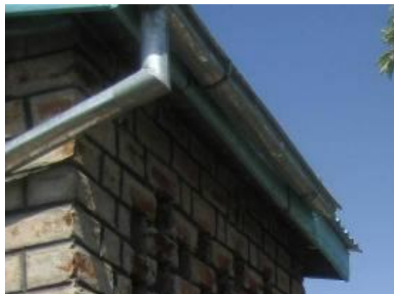
Steel gutter from the back side
