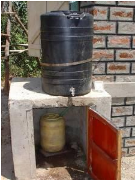
Photo from water tank slab and urine chamber
