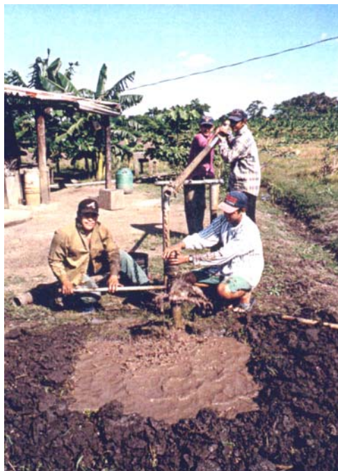
Rota sludge drilling
