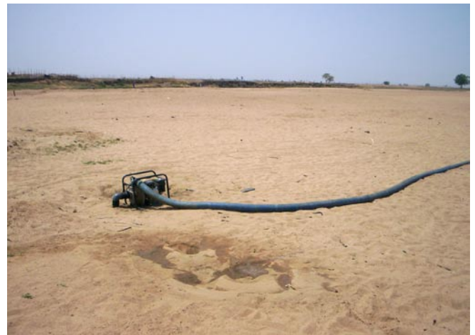
Figure 6 Tubewell fitted with petrol pump on the dry bed of River Faro
