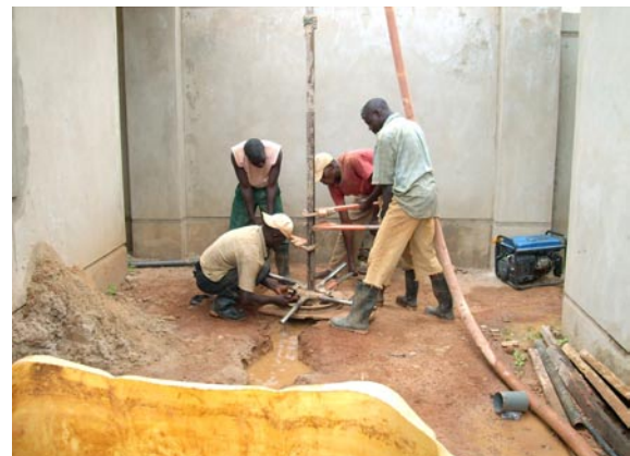
Figure 10 Hand turners work at a private residence
