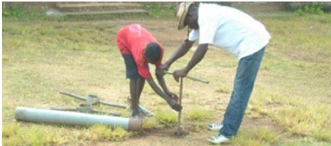
Figure 1 Opening the hole with a hand auger
