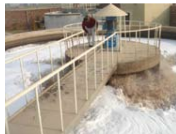
Secondary treatment of tannery waste water
