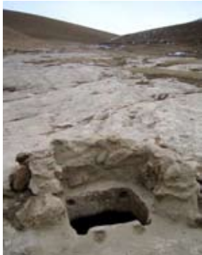
Kanda System. Run-off is collected in a cistern hewn from mountain rock, Afghanistan
