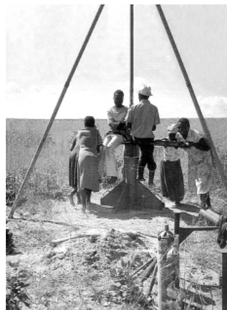
Figure 21 Augering (Note: the men provide the weight and the women provide the labour)
