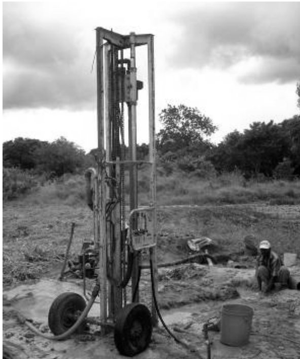
Figure 25 Small Drill Rigs
