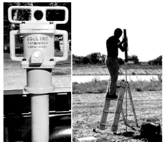
Figure 19 Well Driving
