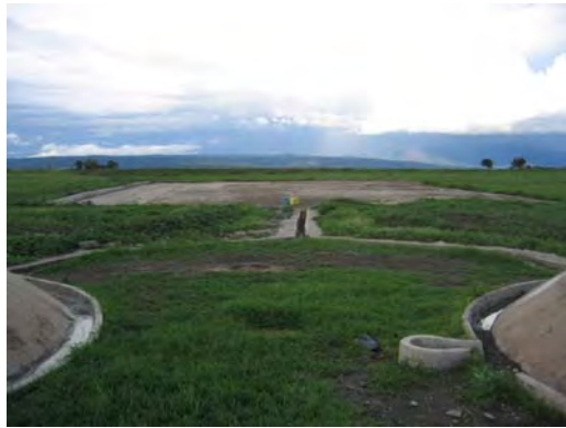
Concrete catchment structure near M'timmoja, Monduli district, Tanzania (from 1945)
